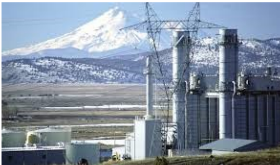
Klamath Falls cogeneration facility Source: Iberdrola Renewables
