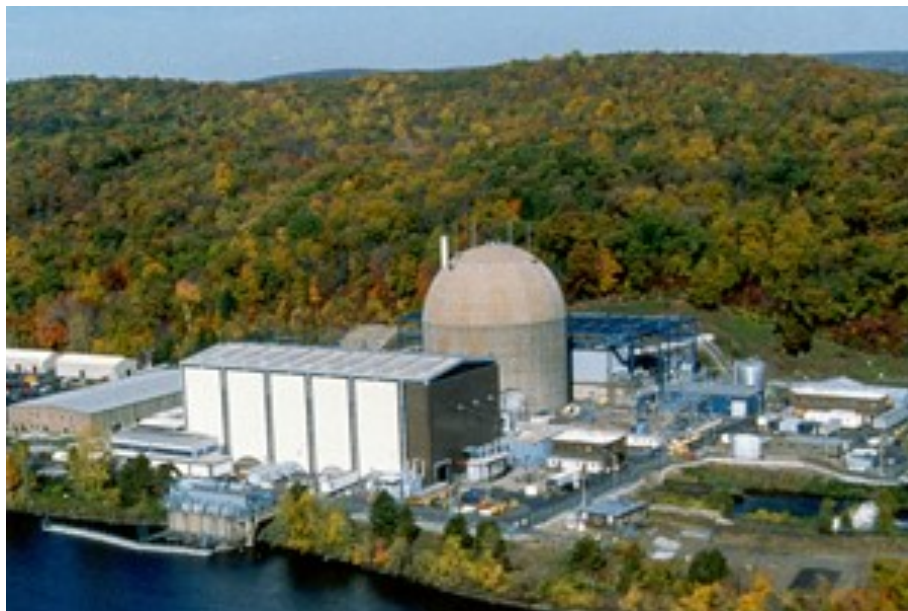
Connecticut Yankee nuclear power plant Source: Nuclear Regulatory Commission
